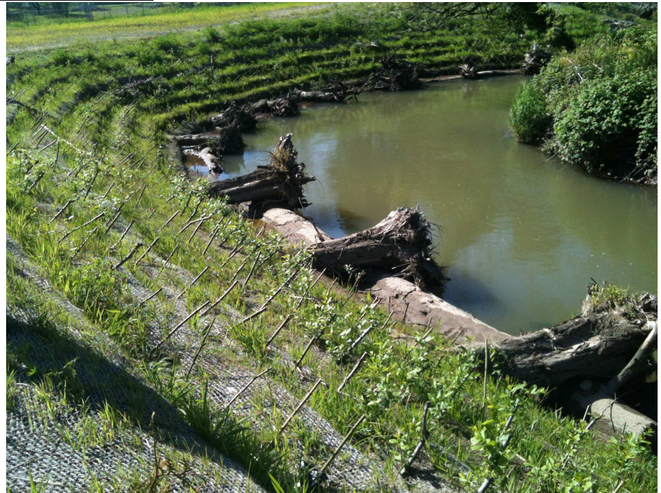
C. Live Log Crib Wall after vegetation
