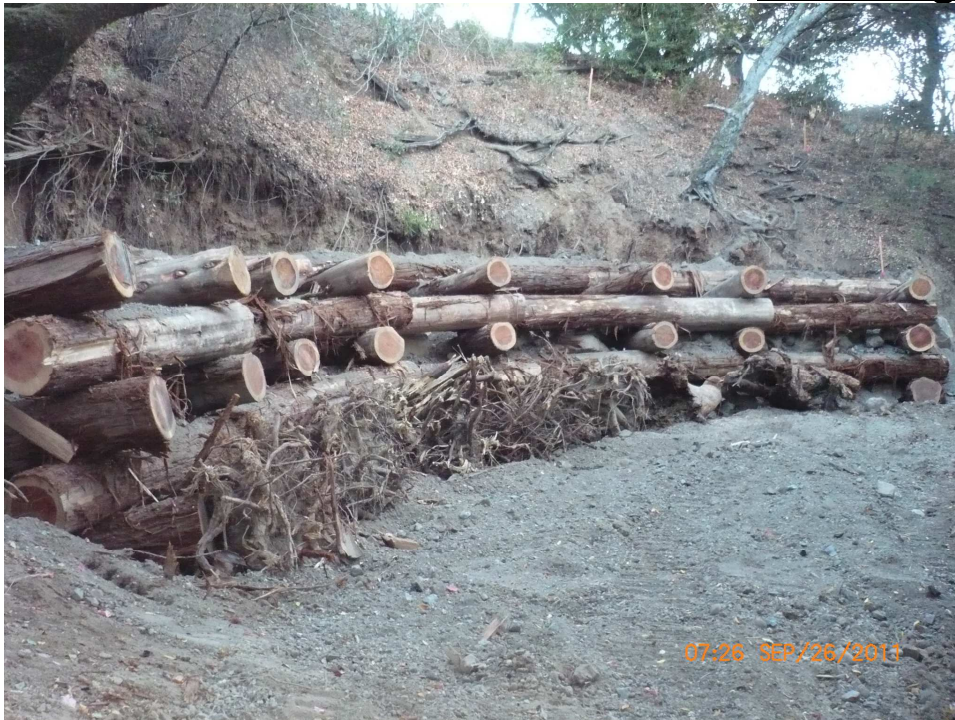
B. Placement of Live Crib Wall
