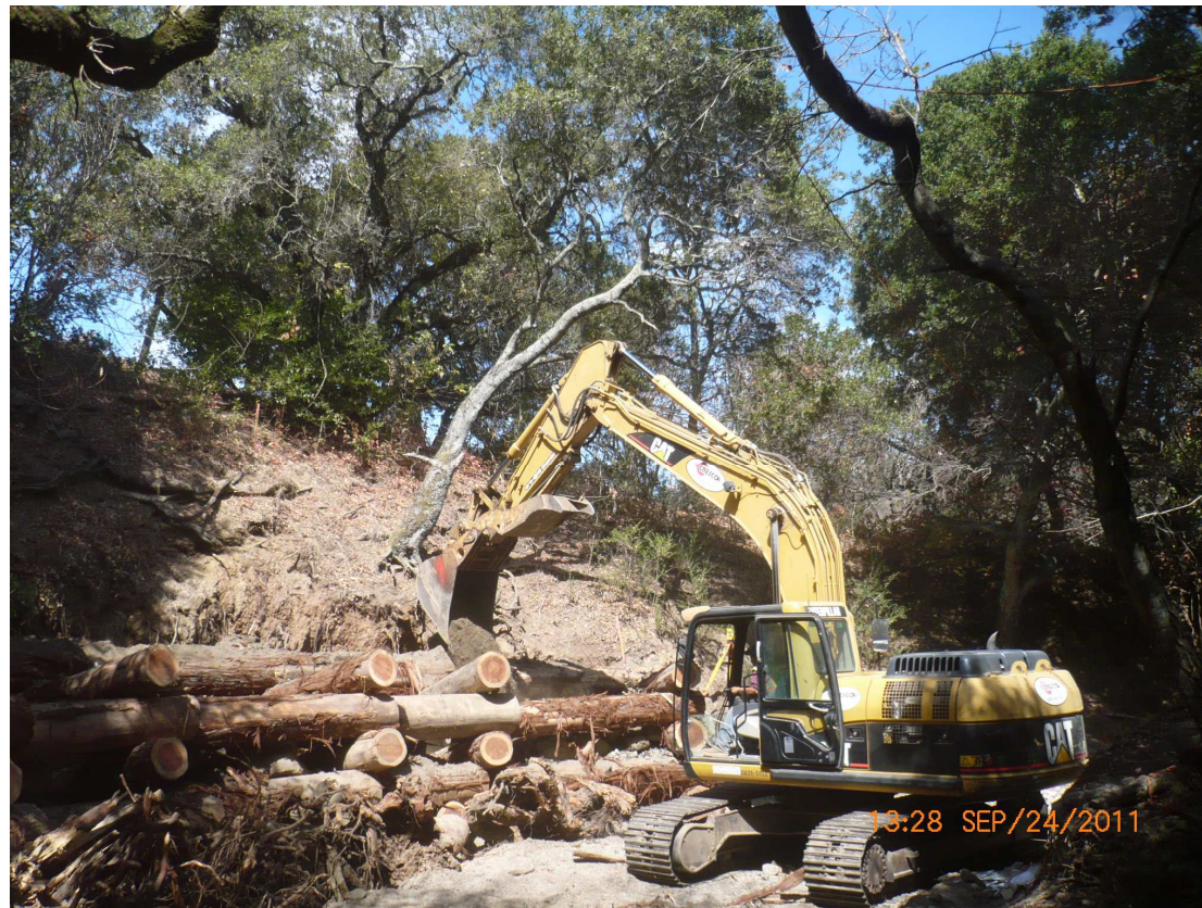
A. Installation of Live Crib Wall
