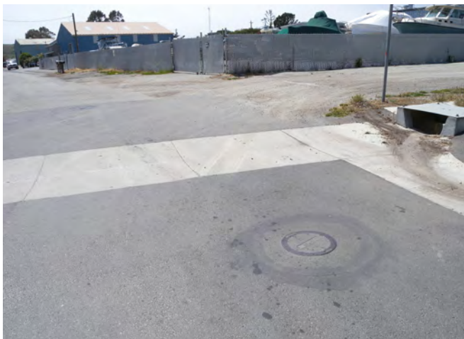
Newly paved streets are lined with concrete swales.
