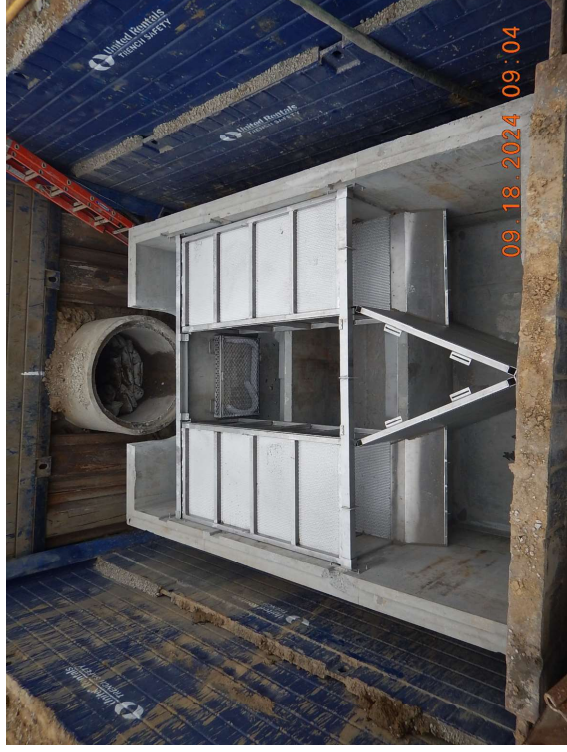
Athlone Terrace Pump Station Trash Capture Device.
