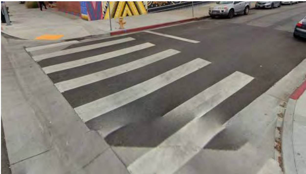
Example of an ADA-compliant curb ramp, high-visibility crosswalk, and advanced stop bar
