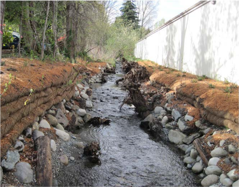
Constructed Creek Realignment and Re-vegetation
