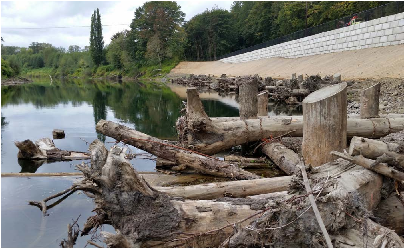
Constructed Vegetated Log Retaining Wall
