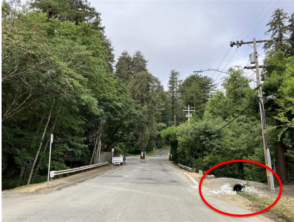
Project Location looking (west) towards Hwy 84 (La Honda Road)
