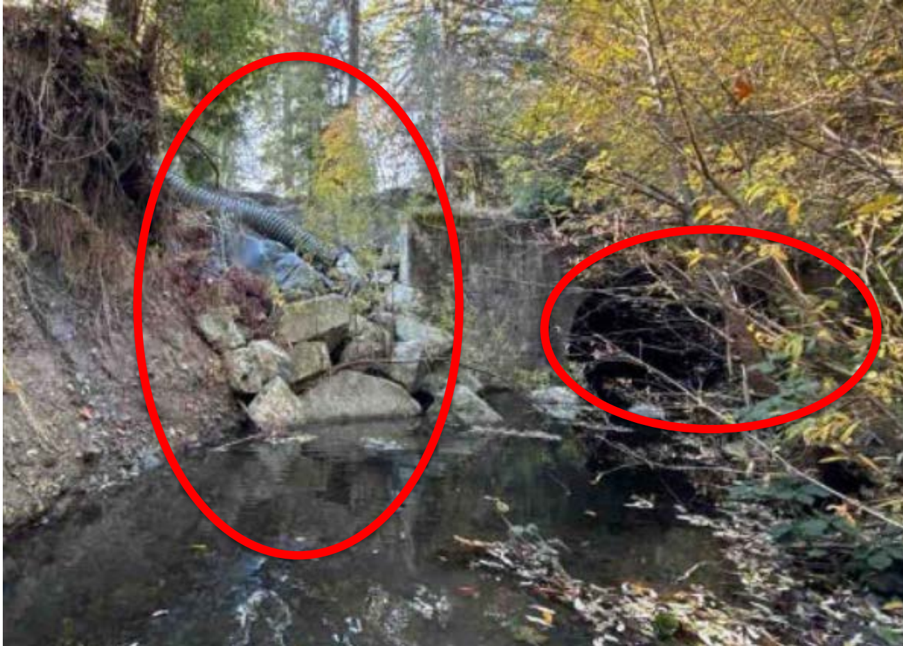
Embankment and Culvert Looking Downstream
