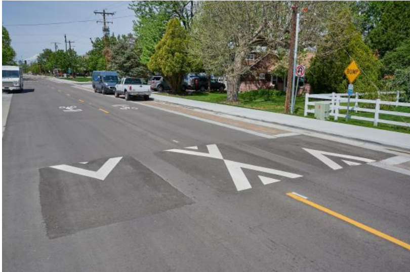
Exhibit A : Asphalt speed hump for two-way traffic with directional striping and gaps for uninhibited passage of emergency vehicles.
