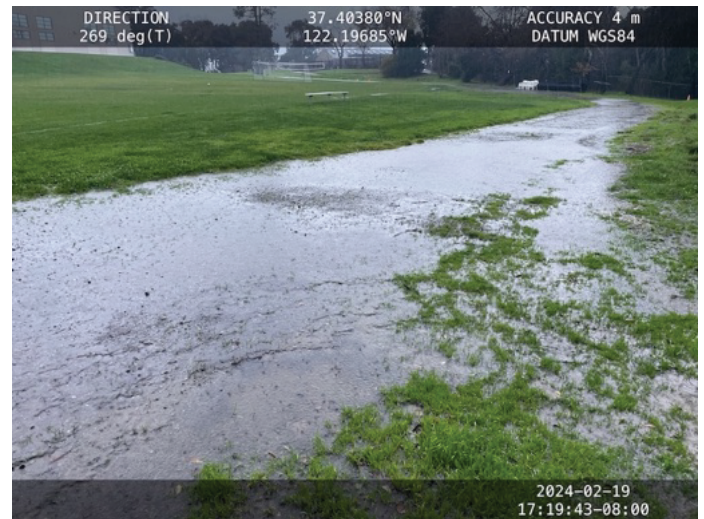
Looking west showing water on access road alongside bioretention basin bypassing both basin and field drain.
