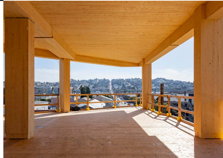
Right: CLT panels are lifted into place and then secured.
