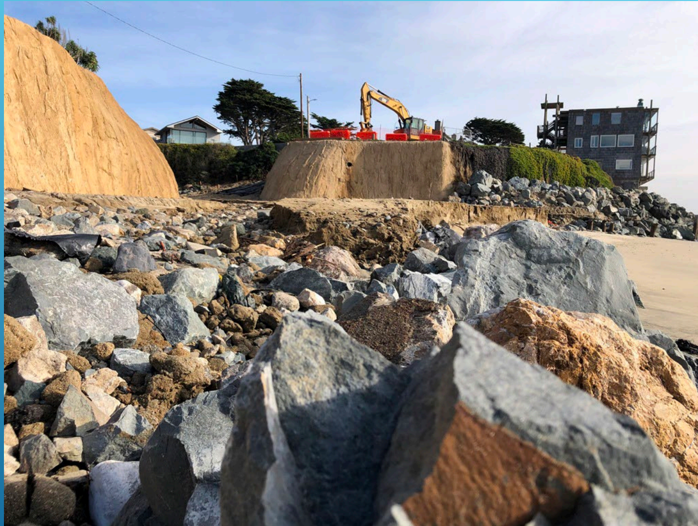
MIRADA ROAD PEDESTRIAN BRIDGE SHOTCRETE WALLS COMPLETED
