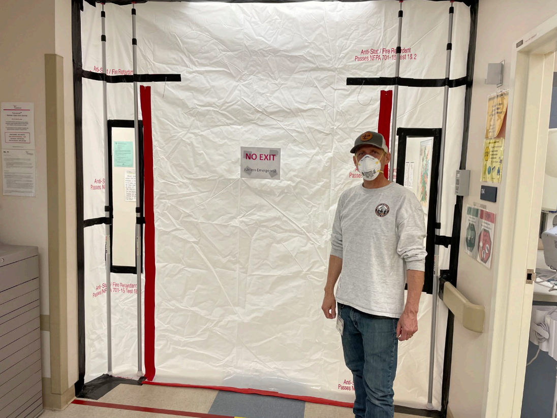
CONTAINMENT SETUP AT SMMC
