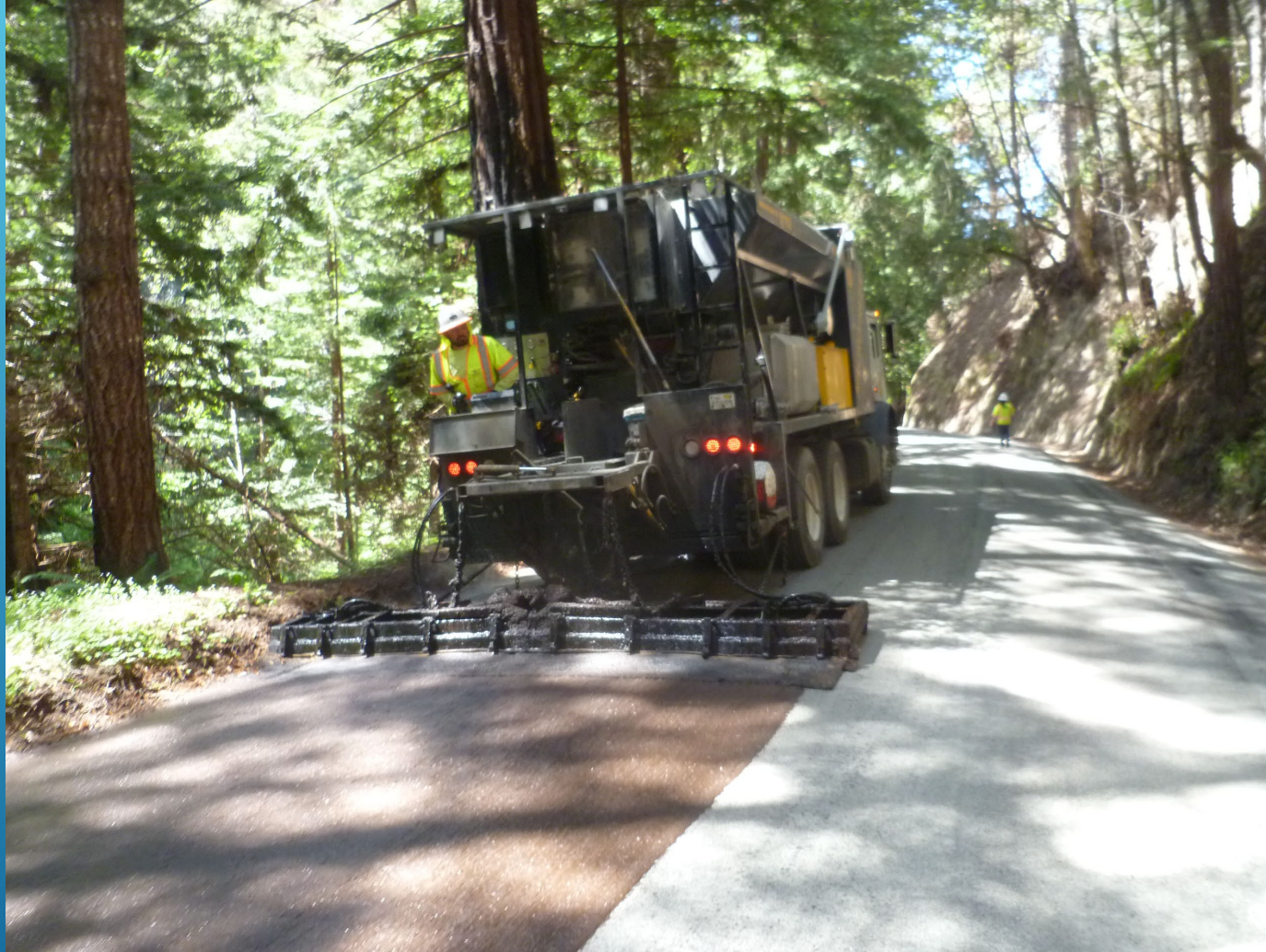
MICROSURFACING APPLICATION ON GAZOS ROAD
