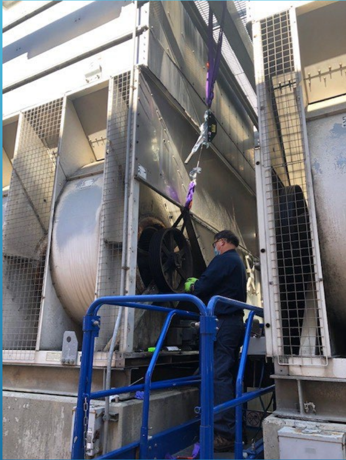
COOLING TOWER REPAIR
