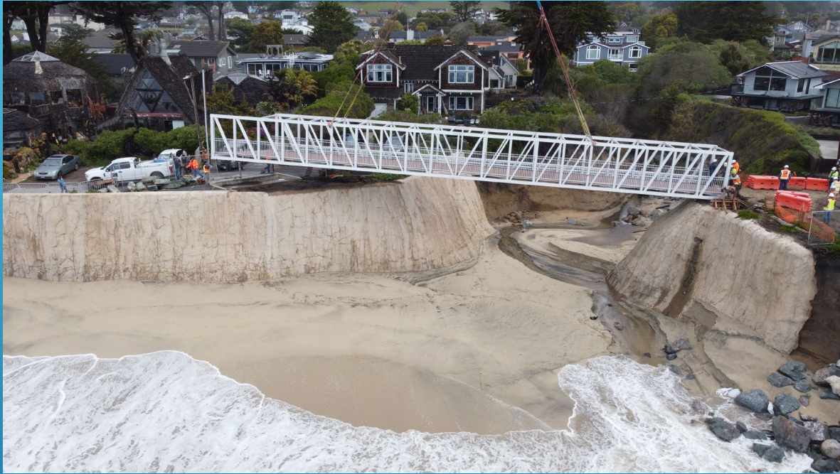
INSTALLATION OF THE MIRADA ROAD PEDESTRIAN BRIDGE ON MAY 4, 2023
