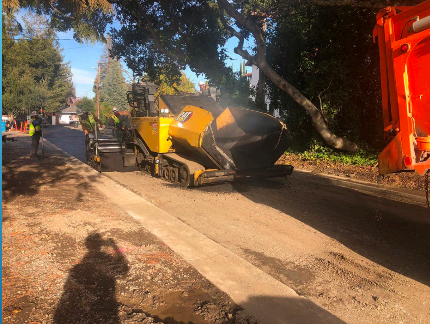
PAVING OF ENCINA AVE IN THE NORTH FAIR OAKS AREA
