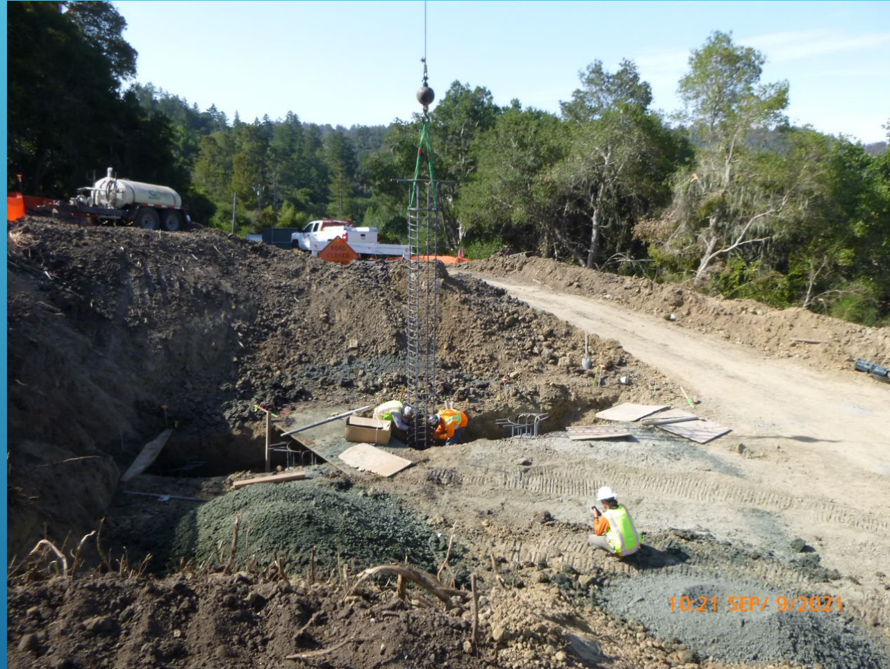
SCENIC DRIVE RECONSTRUCTION INSTALLATION OF STEEL CAGE FOR RETAINING WALL PILE
