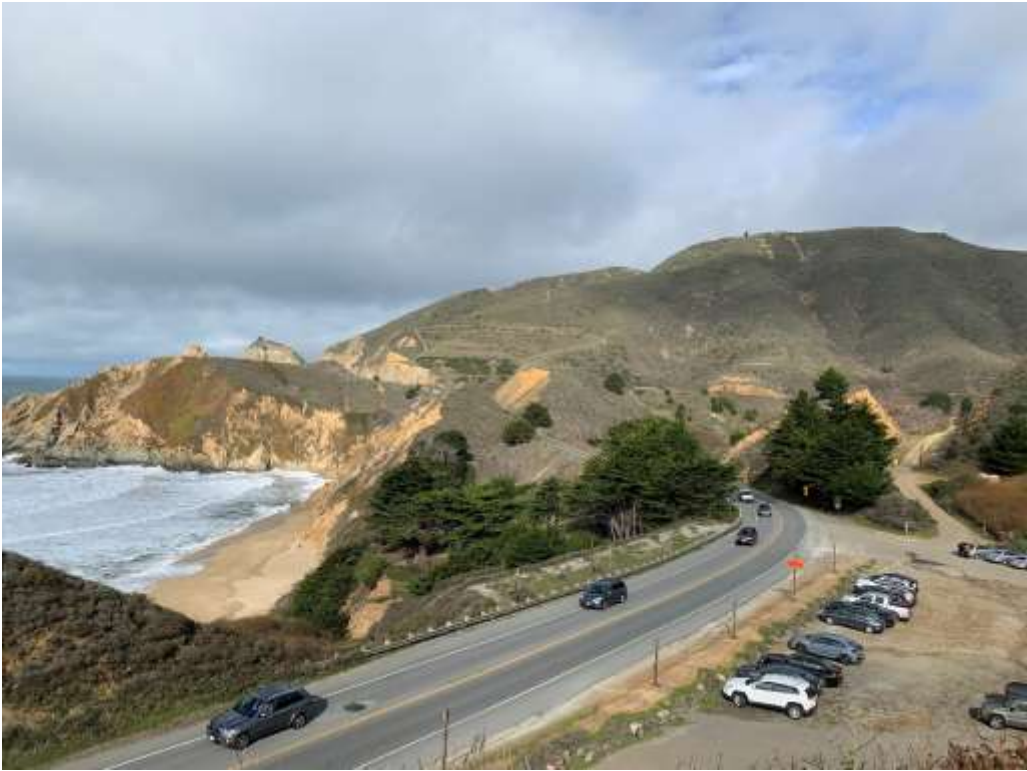
Parking lot with no marked crossing of Highway 1 to reach Gray Whale Cove
