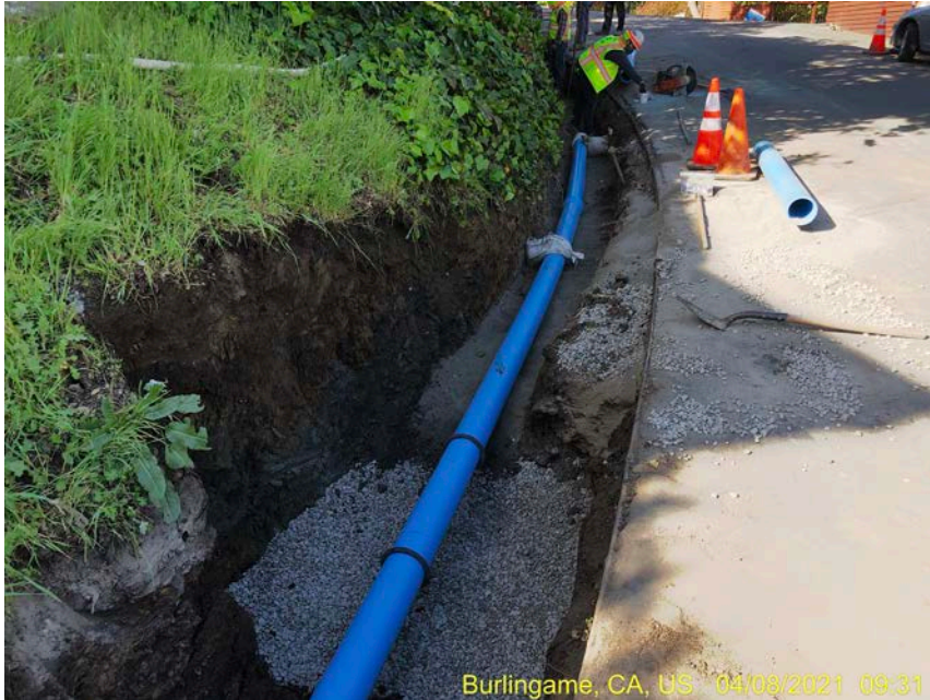
→ Pipe Laying and Lateral Connection
