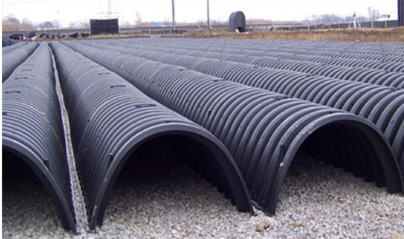
Figure 5.1. Installation of subsurface storage for a Regional Project (Source: Conteches.com)
