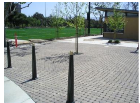
Figure 1.10. Permeable Interlocking Concrete Pavers, Mayfield Playing Fields, Palo Alto.
