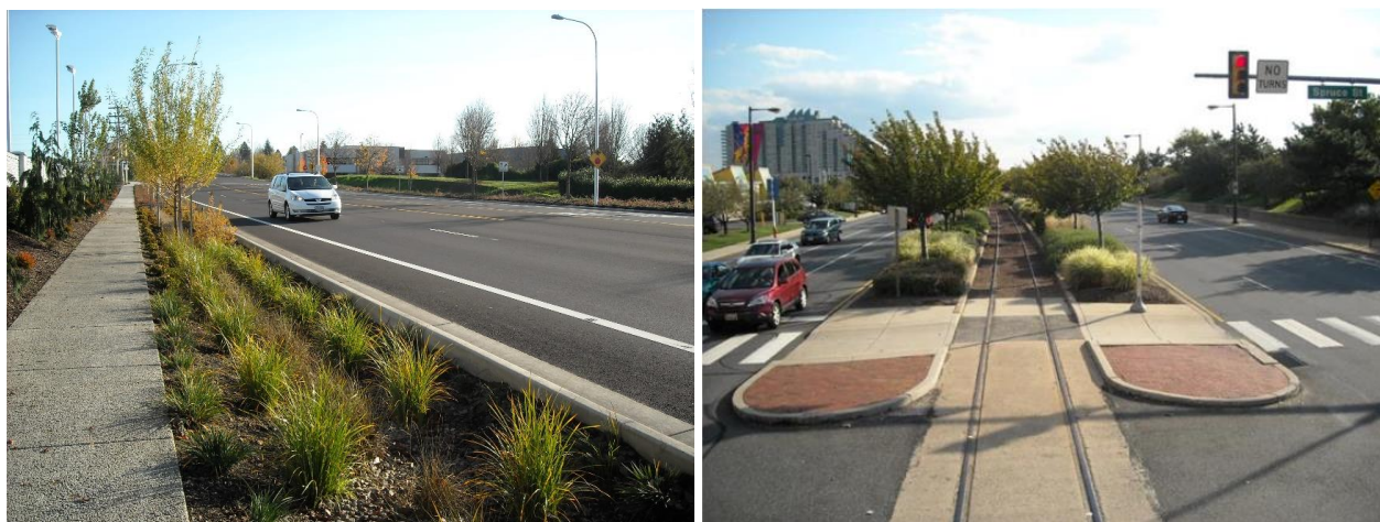
Figure 5.3. Green Street example, Brisbane (left). Street design featuring multiple transportation options (right). (Source: SMCWPPP)
