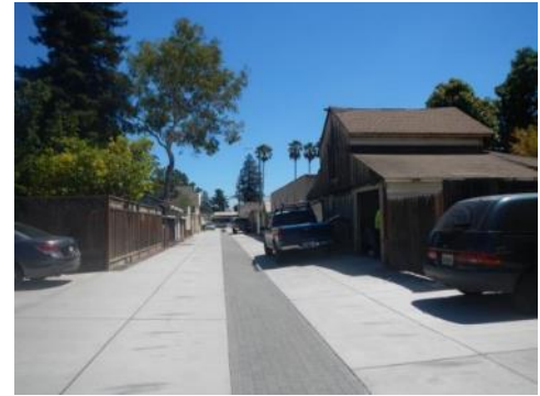
Figure 1.11. Infiltration trench, San Jose. (Source: City of San Jose)
