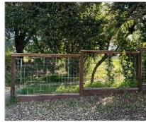
hogwire panel fence 5' or 6' tall, 2x4 frame with 2x6 top, 4x4 pressure treated post and 1x1 picture frame around wire panel
