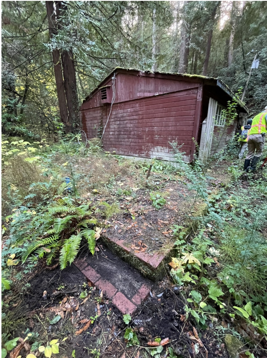
Photo 18: Cabin Site – Honeymoon Cottage Foundation
