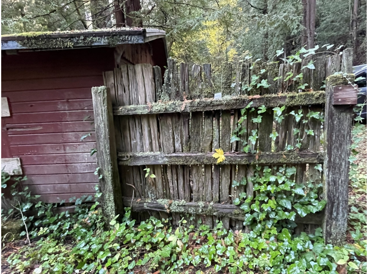
Photo 17: Cabin Site – Fence at Garage
