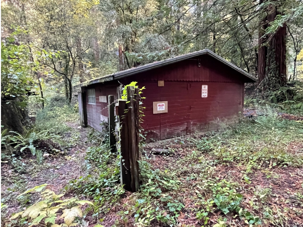
Photo 16: Cabin Site – West Elevation of Garage
