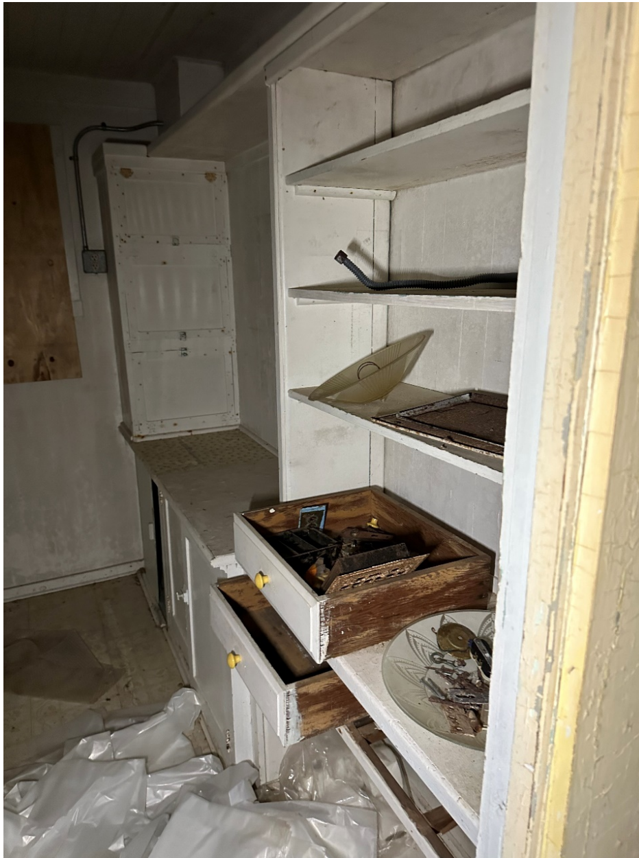
Photo 11: Cabin Interior – Pantry Cupboards
