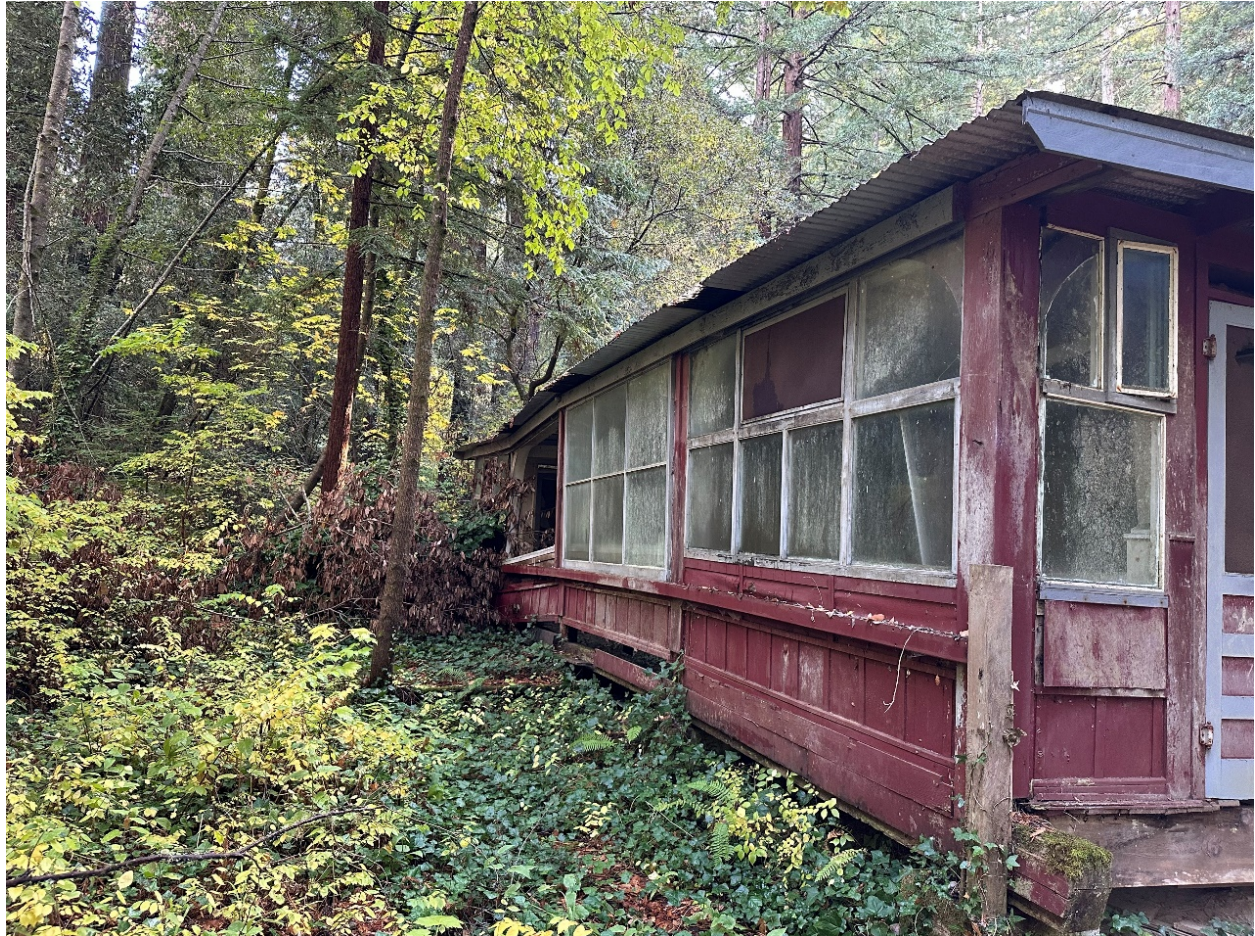
Photo 4: Cabin Exterior – East Elevation from Northeast Corner
