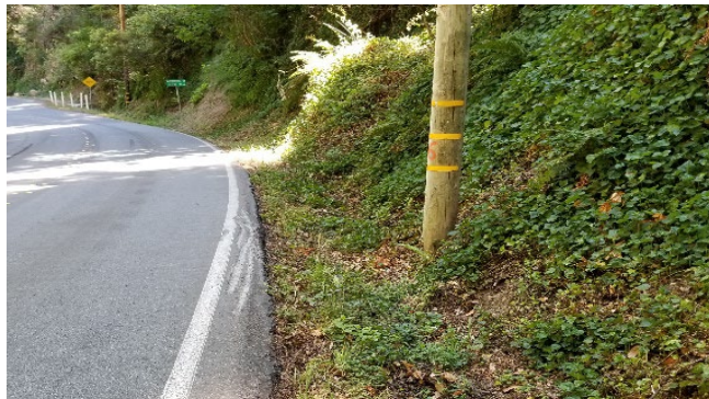
Photos 4 & 5 Loma Mar Section-Top photo 4: some recovery area on approach to curve, shoulder widening. Bottom photo 5: fixed object, no all-weather shoulder, edge drop-off. Photo credit: FHWA
