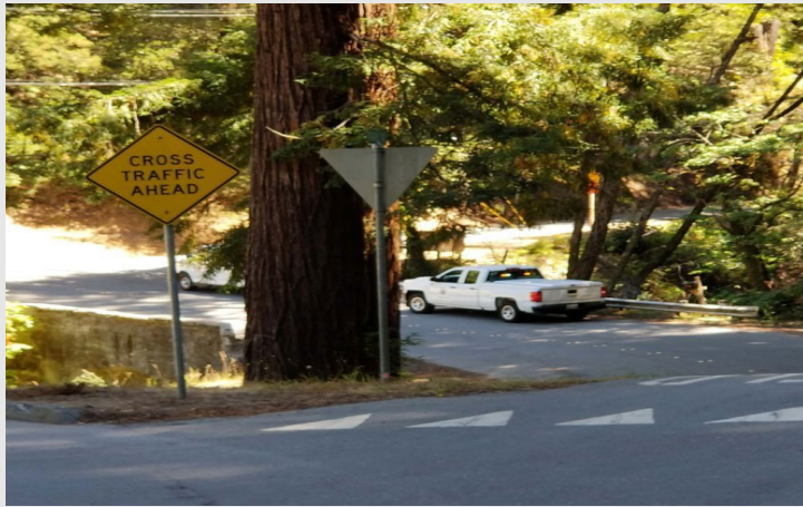
(Photo credit FHWA ) View of connector road to Alpine Road just downstream of point of curve of PCR (EB)
