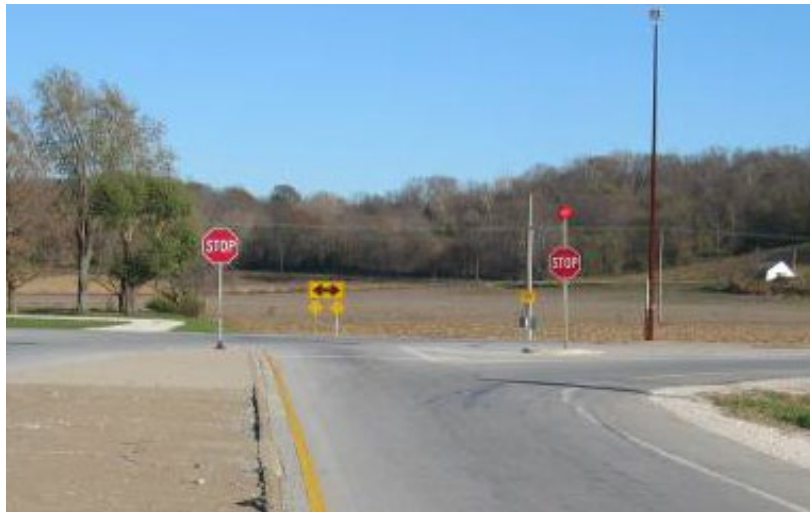
Photo 3 - Example of a supplemental STOP sign mounted on left in a splitter island. Location and photo credit unknown
