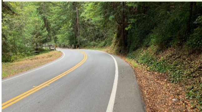
Photos 4 & 5 Loma Mar Section-Top photo 4: some recovery area on approach to curve, shoulder widening. Bottom photo 5: fixed object, no all-weather shoulder, edge drop-off. Photo credit: FHWA
